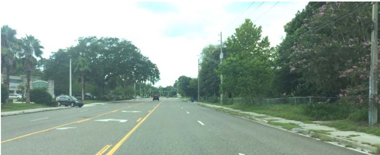
Facing west along New Berlin Rd.
